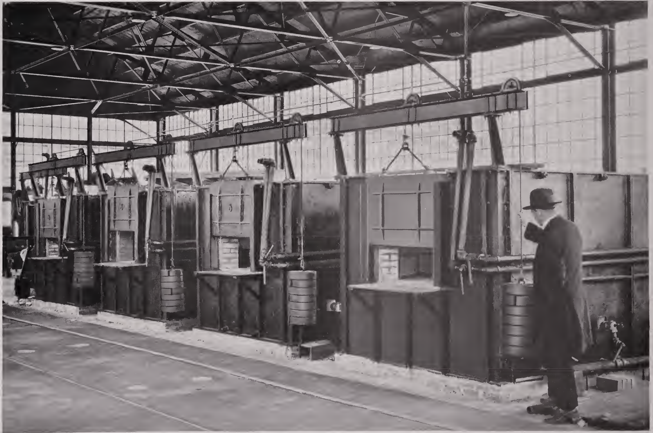
ONE OF THE BATTERIES OF HEAT TREATING OVENS
